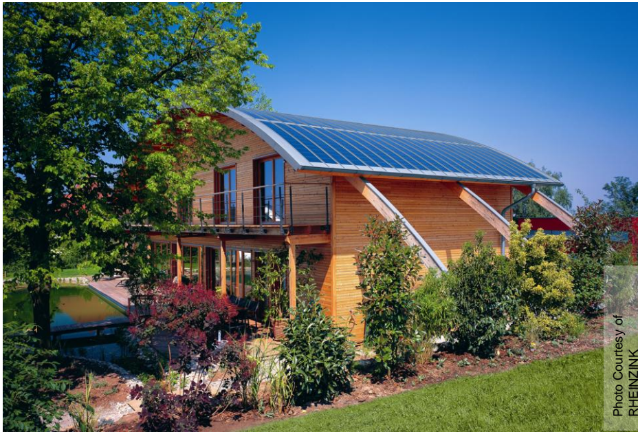
5.6 kW residential installation in Germany
