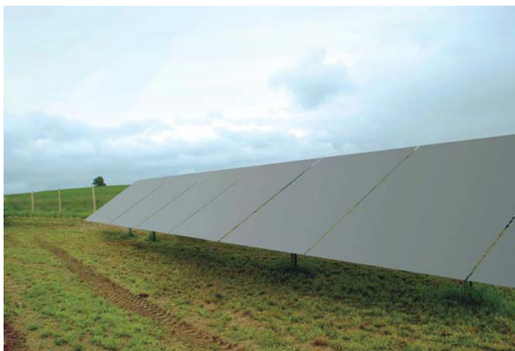
Solar, Big and Lean: An installation in Germany of thin-film solar panels, each measuring 18.7 square feet. | Photograph Courtesy of Applied Materials
