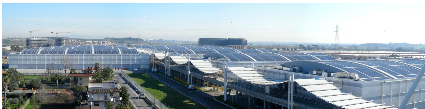
Iscom & Green Utility Rome, Italy 1400 kWp
