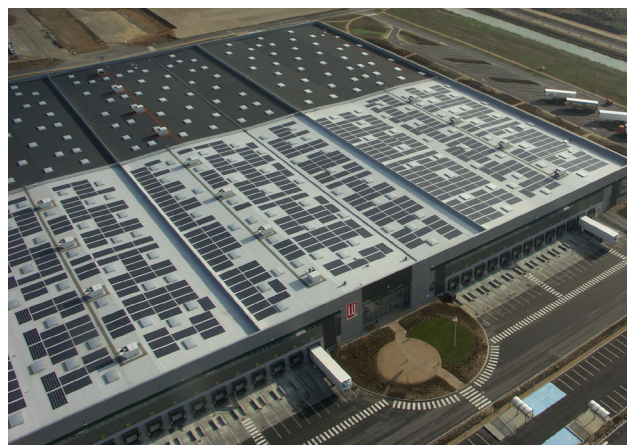
Solar Integrated Technologies Moissy-Cramayel, France 446 kWp
