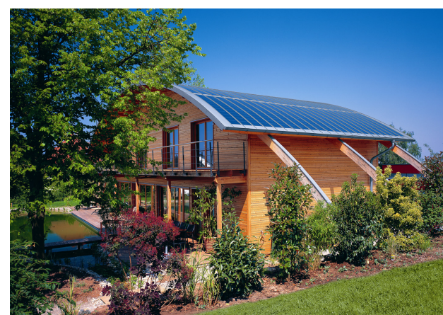
RHEINZINK Heilbronn, Germany 5,6 kWp
