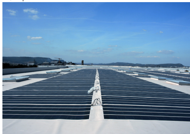
Solar Integrated Technologies Laudun L'Audoise, France 1393 kWp
